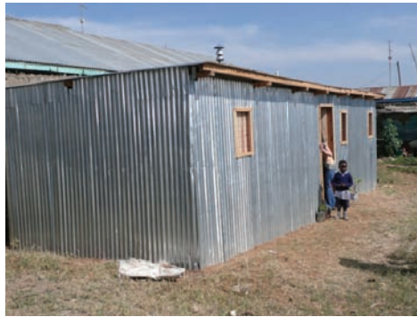
A child stands outside the door to his new home built by the Joliet Diocesan mission volunteers during their visit in September.
